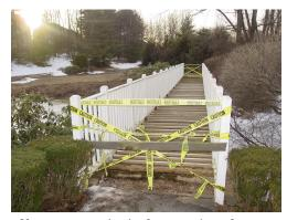
In addition, the bridge between the pool and the parking lot is undergoing some major repair. The bridge deck, which was sorely splintered and not holding stain any longer, is being replaced by Trex, a material that resists damage from moisture and insects and provides excellent traction even when wet. This is a one-time expenditure and will provide a low maintenance solution for the bridge.
