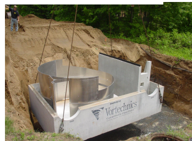
Vortechnic Unit being installed in 2006
